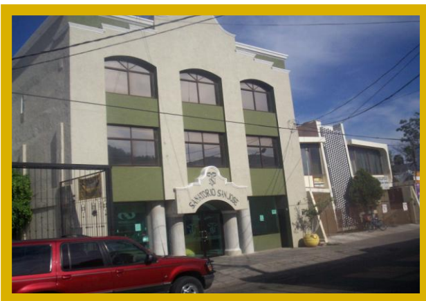
HOSPITAL SAN JOSE
